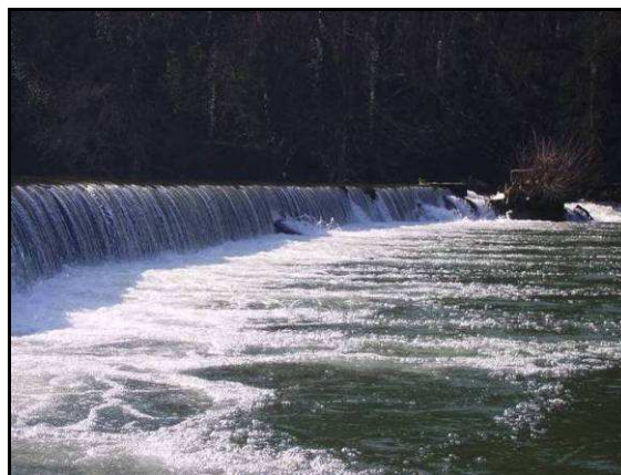
FIG. 83 – Açude 2 (41°32'17.8" N, 008°34'43.5"W)
