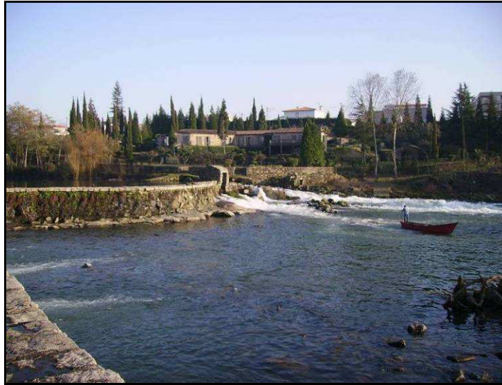
FIG. 89 – Açude 6 (41°31'16.8" N, 008°38'09.0" W)
