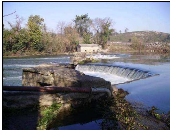
FIG. 82 – Açude 1 (41°32'45.7" N, 008°33'12.2" W)
