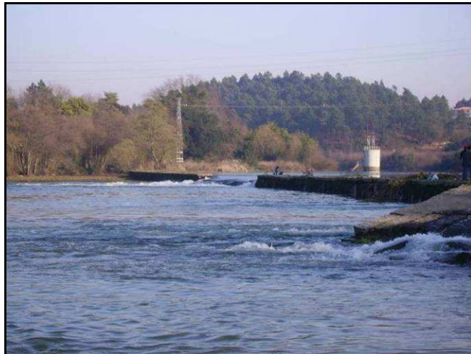
FIG. 86 – Açude 4 (41°31'37.5" N, 008°36'57.8" W)
