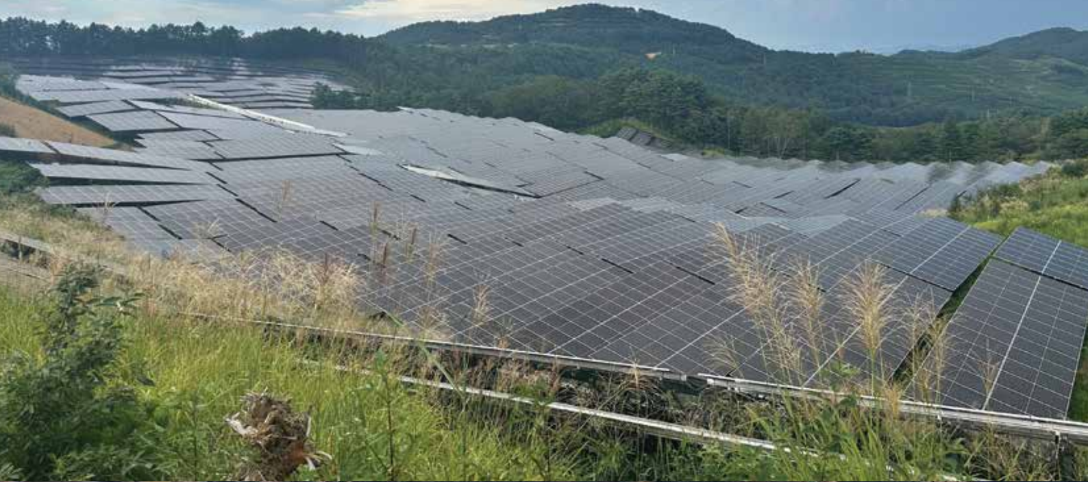
Motoyoshi Solar Farm 28 MWp Miyagi Prefecture, Japan ※Illustrative rendering of the site
