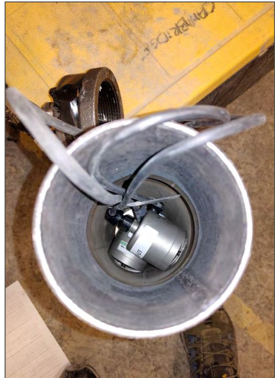
Photograph 2: Uniaxial accelerometers (longitudinal and transverse direction) bolted to the steel .
