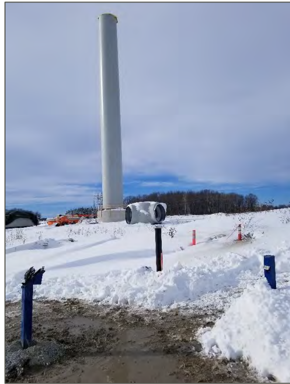
Photographs 5 and 6: “Mock Well” steel casing installed and protruding above ground surface at one turbine site (left); Mock Well casing location with respect a wind turbine structure (right).
