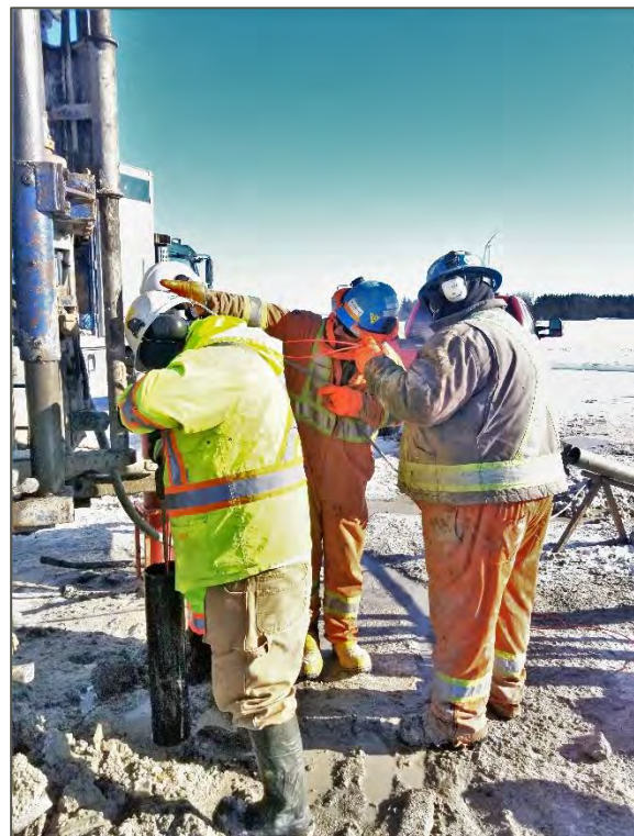
Photograph 3: Assembled protective steel casings containing sets of accelerometers (3 orthogonal directions); Installation of protective steel casing containing a set of accelerometers (3 orthogonal directions) (right)
