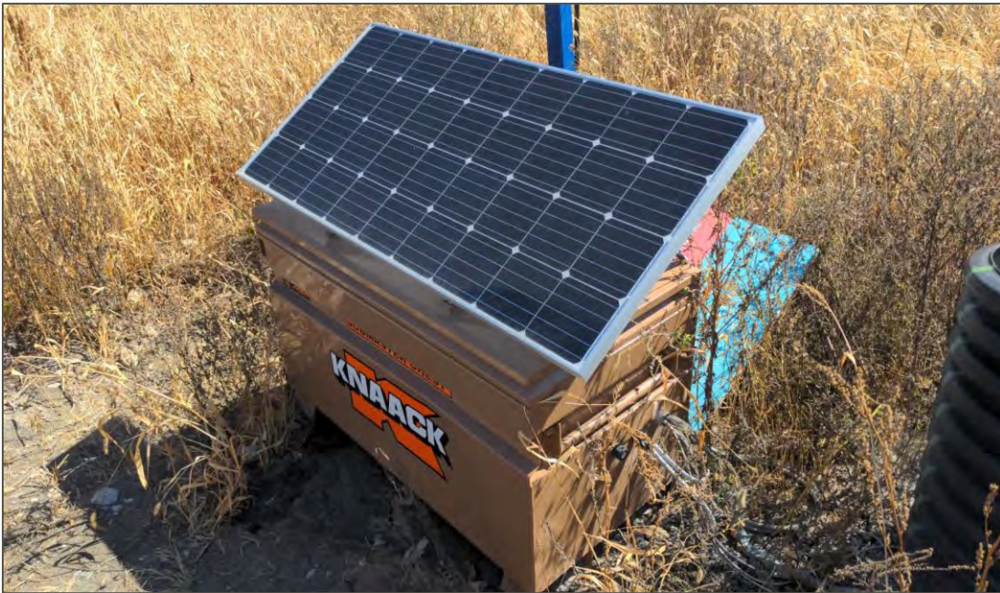
Photograph 7: T10/11 Mock Well protective steel box. Note lid-mounted solar panel arrangement.
