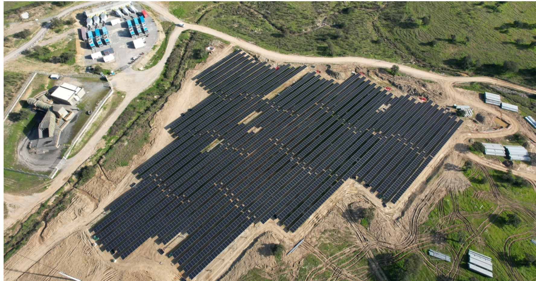
Image: Portugal's largest self-consumption solar plant, developed in partnership with Somincor.
