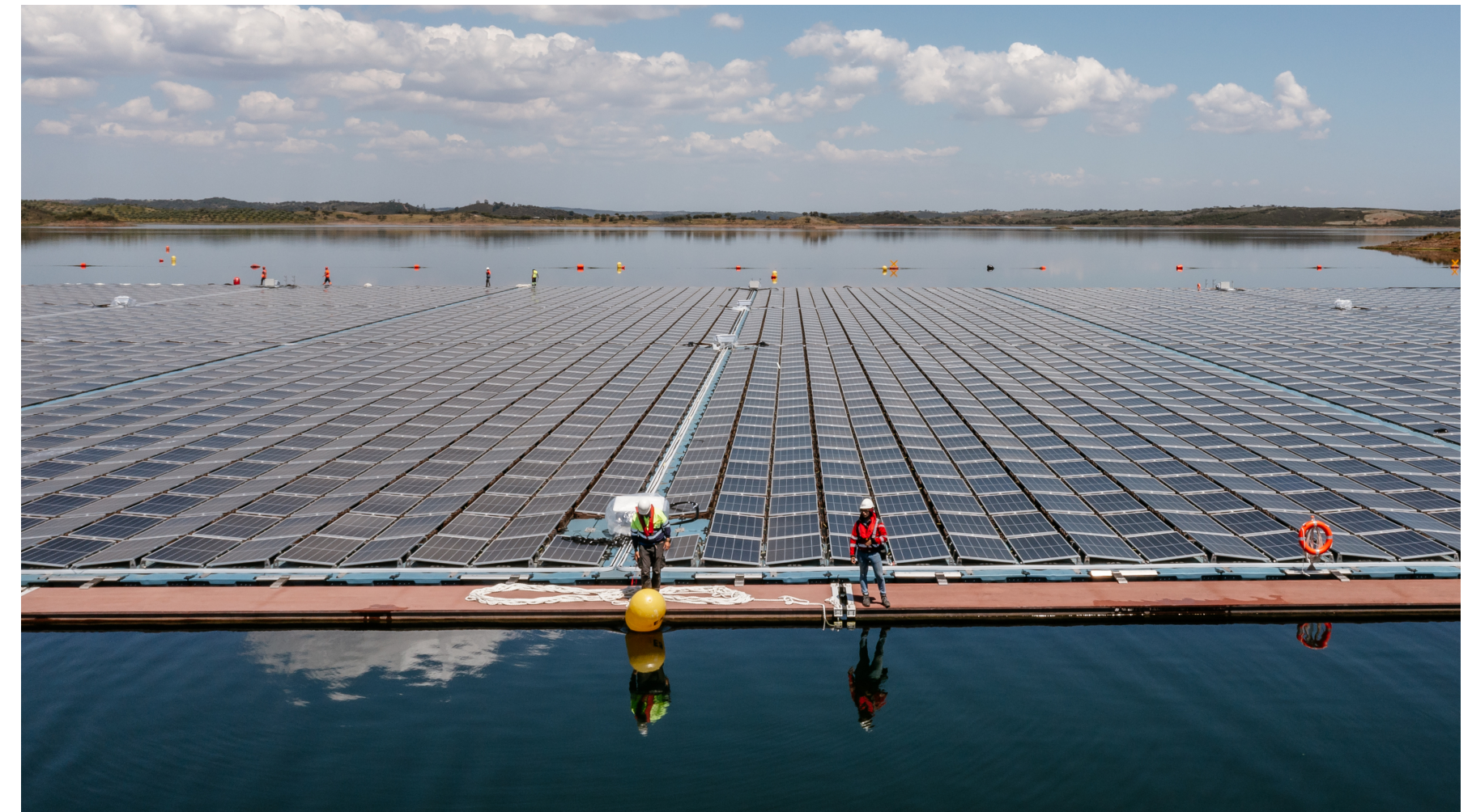
Image: Alqueva Hybrid Park, floating solar generation integrated with hydropower and battery storage at a dam reservoir in Portugal.
