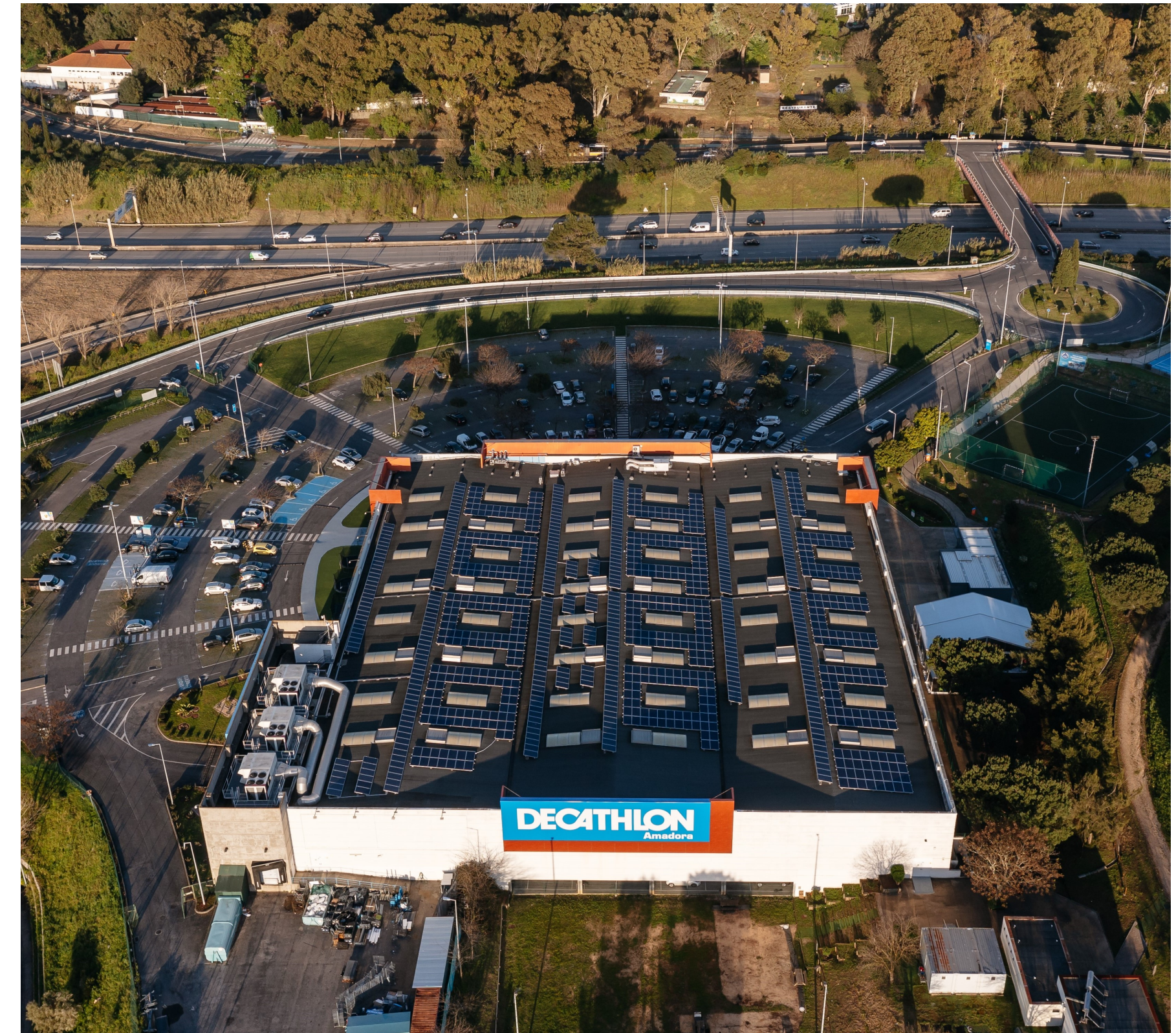
Image: On-site solar photovoltaic installation for a business customer, enabling renewable energy generation and a reduced carbon footprint.
