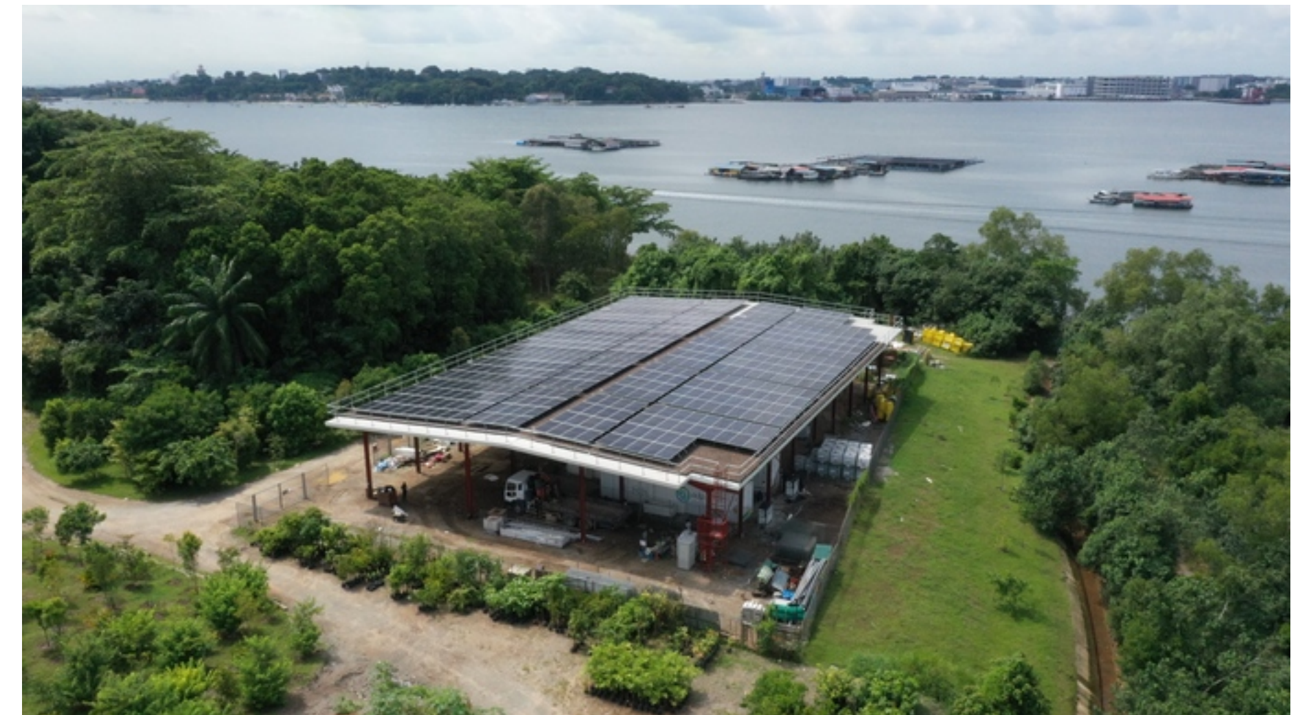
Image: Pulau Ubin Green Microgrid, Singapore: hybrid renewable energy solution combining solar generation and battery energy storage to support a more resilient and sustainable energy supply on the island.
