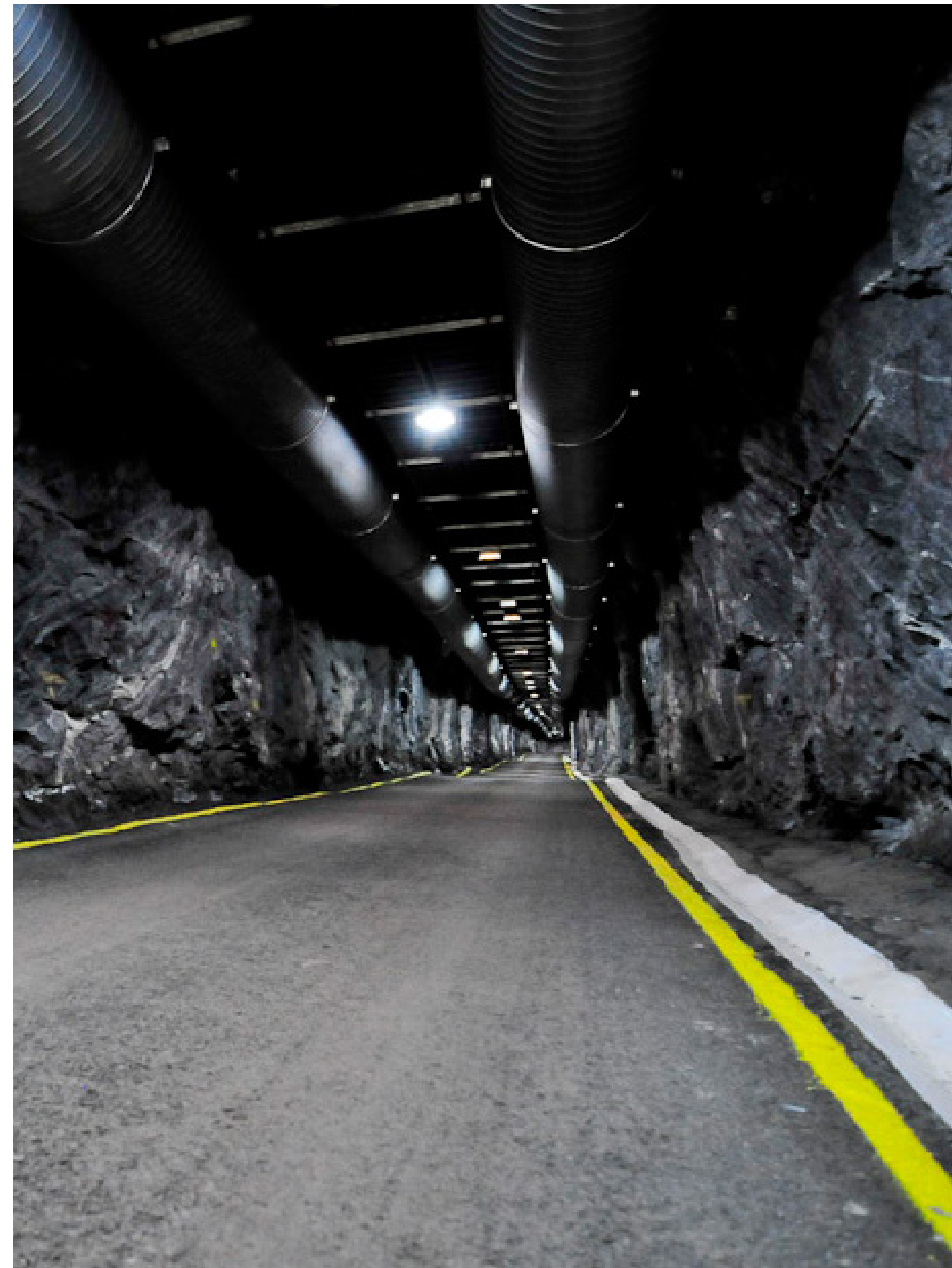
São João SMALL HYDROELECTRIC PLANT (ES)
