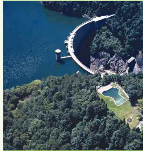
Caniçada Hydro Power Plant
