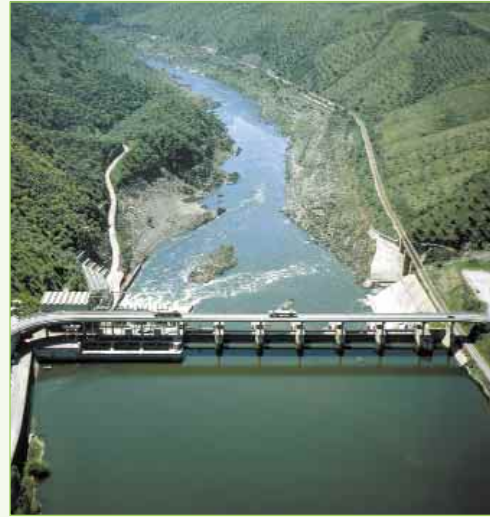
Fratel Hydro Power Plant
