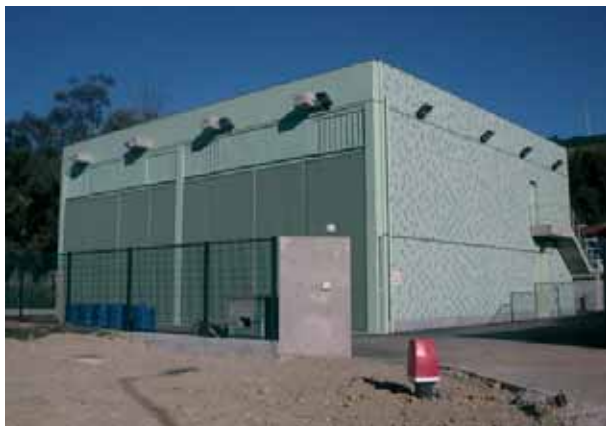
New HV/MV substation in Amadora
