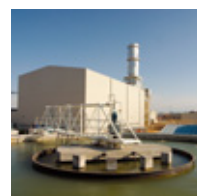
Castejón Combined Cycle Power Station
